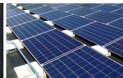
Fast install: 15 men install .93 MW panels, racks & ballast per week
